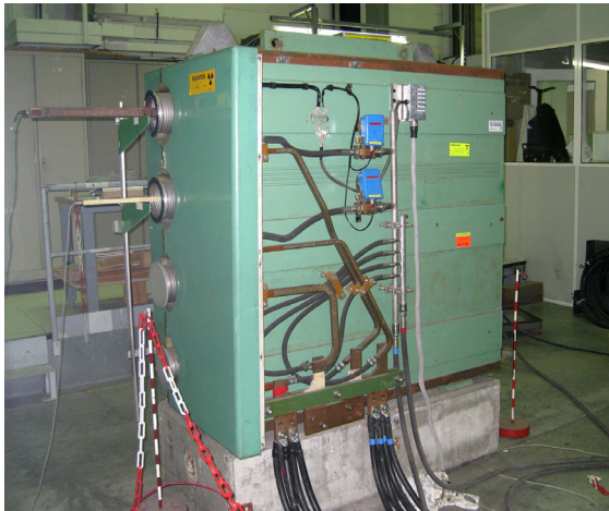
Figure 1: Booster main magnet undergoing tests for operation at 2 GeV.
