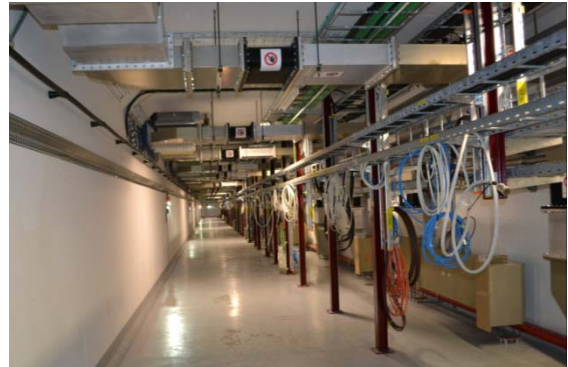
Figure 7: Linac4 tunnel (August 2012).
